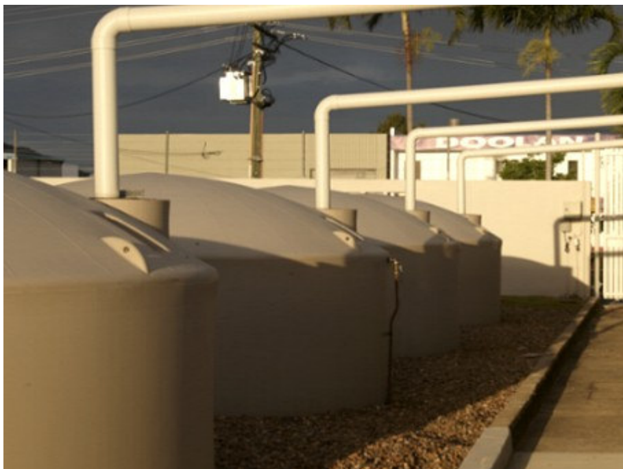
Outside, 100,000 litres of water tanks collect rainwater from the roof. These tanks were manufactured in Townsville.
